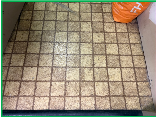
11 2nd Floor; Storage Room Brown Vinyl Sheet Flooring
